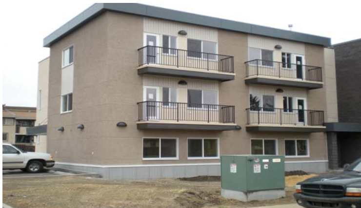
River Heights Addition
